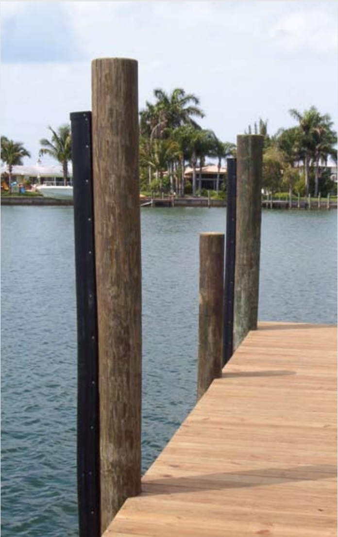
Black Flexmaster bumpers installed on dock pilings (Available in black or white)
