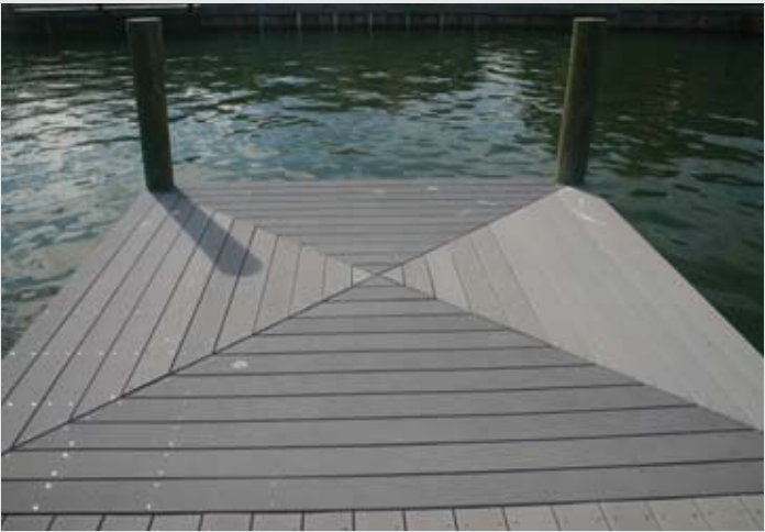
Custom carpentry using composite decking
