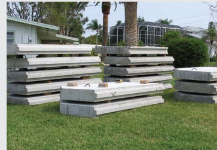
Prefabricated seawall panels ready for installation
