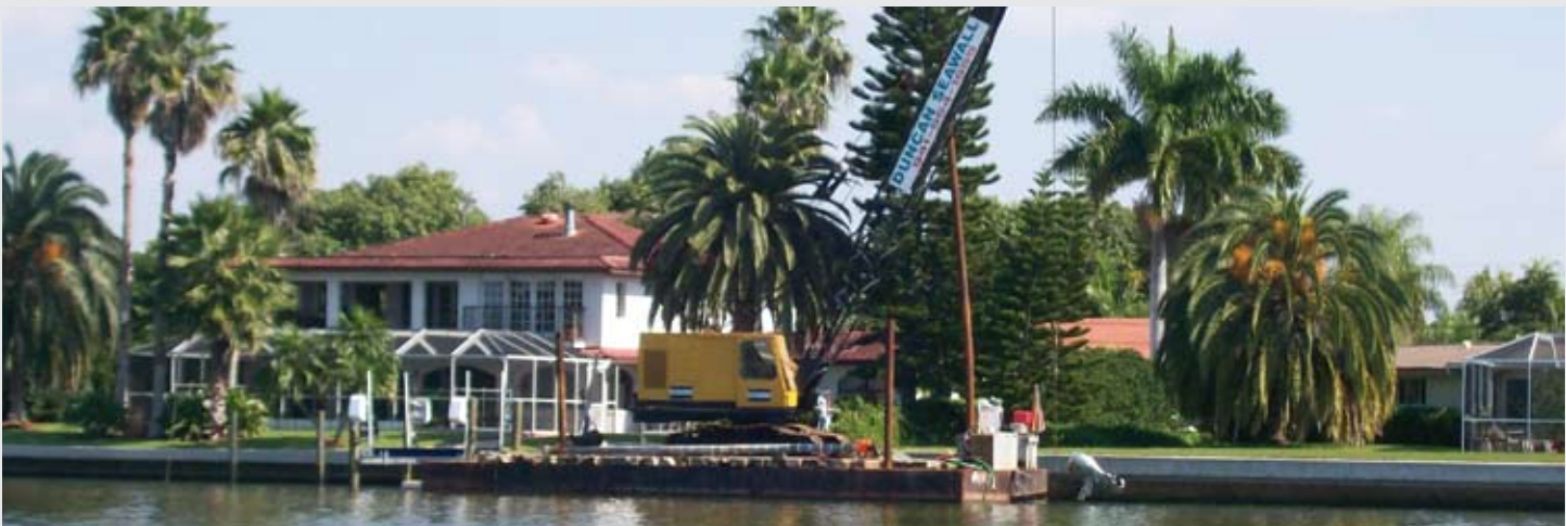
Pile punching crane barge for punching piles into rock
