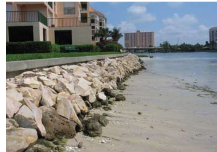
12" – 24" rock installed in front of an existing concrete wall
