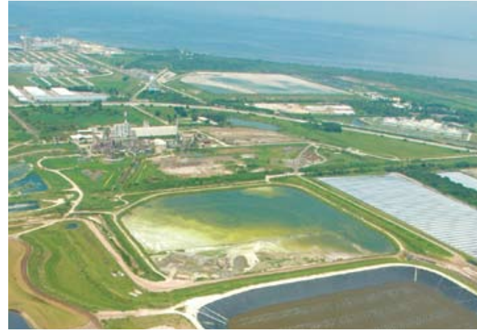
Dewatering cell for hydraulic dredging
