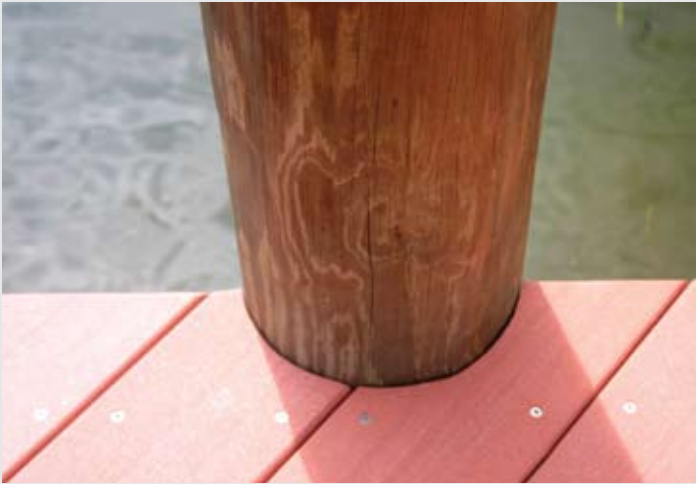
Precision carpentry around dock pilings
