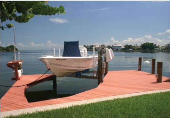
Custom configured marginal dock with composite decking and 7,000 lb. capacity beamless lift
