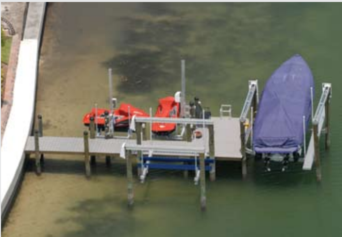
Access and terminal dock with two 10,000 lb. capacity conventional lifts and two aluminum PWC lifts
