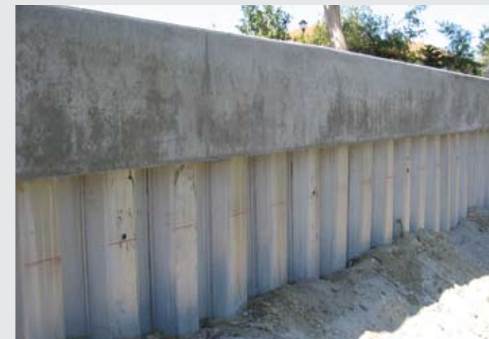
Aluminum wall with concrete cap
