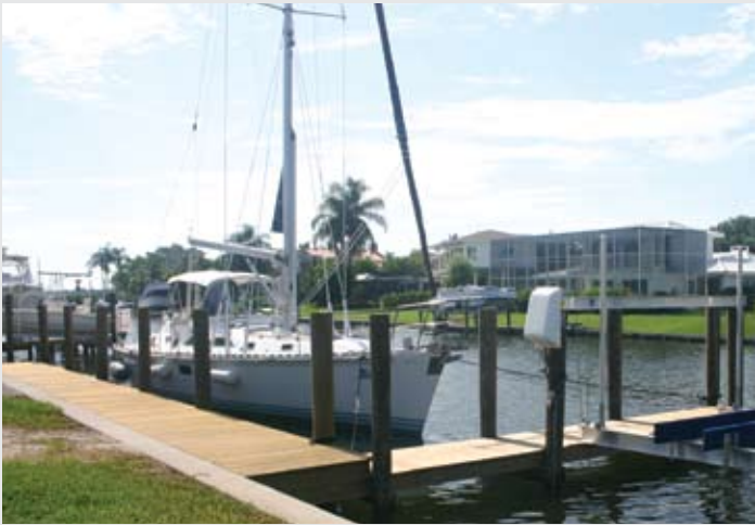
5' x 50' marginal dock with a 4' x 28' finger pier constructed with Pro Deck pressure treated timbers and 7,000 lb. capacity conventional lift
