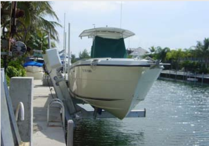
10,000 lb. capacity elevator lift mounted to seawall
