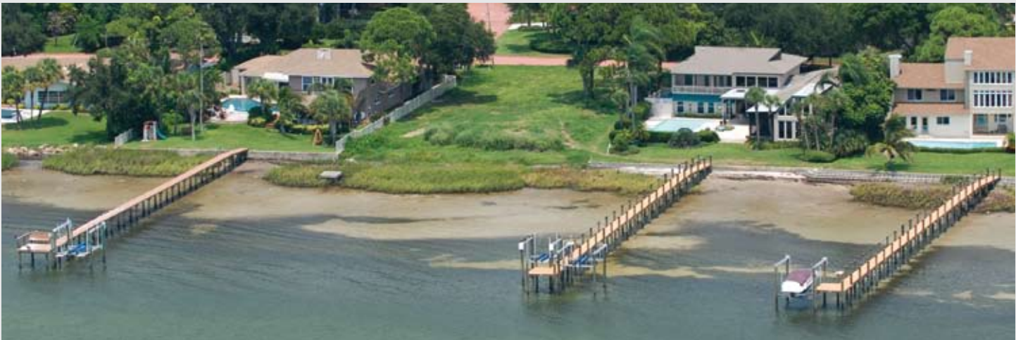
Three 200' long access and terminal docks with composite decking and various lift types and sizes
