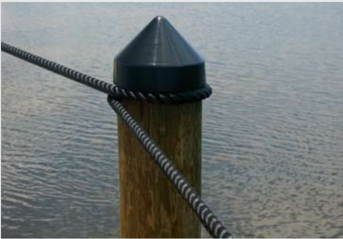
Black piling cap with rope railing
