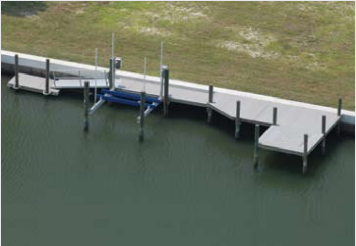
Custom configured marginal dock with 10,000 lb. capacity beamless lift and floating platform
