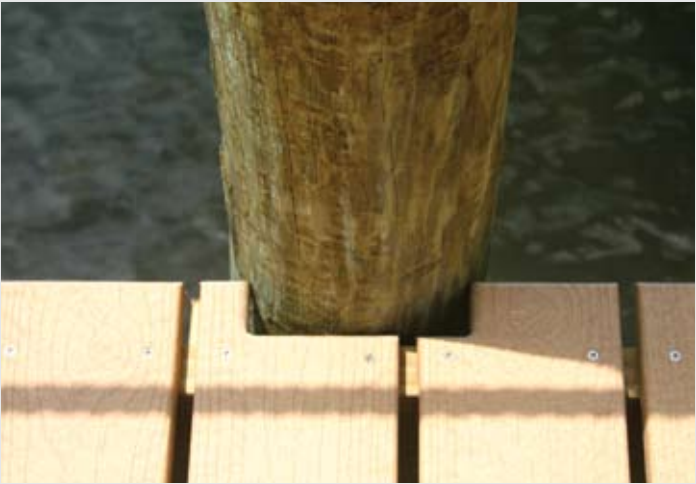
Square cutting around pilings
