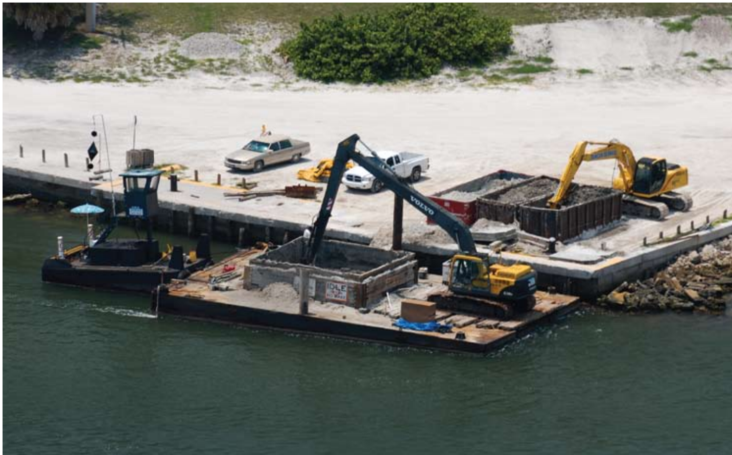
Off-loading site for a barge based mechanical dredge
