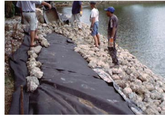
Nylon filter cloth placed over the shoreline prior to rock placement
