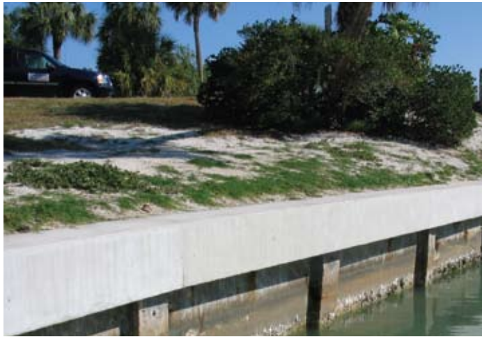
New cap and tiebacks installed on existing concrete seawall
