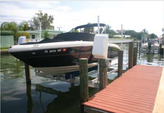
5' x 20' marginal dock with composite decking and a 10,000 lb. capacity conventional lift
