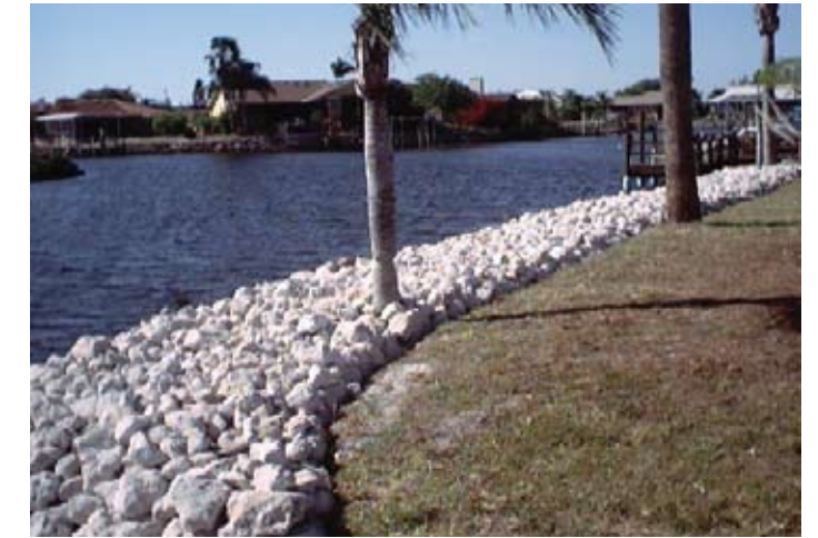
6" – 18" rock installed along graded shoreline
