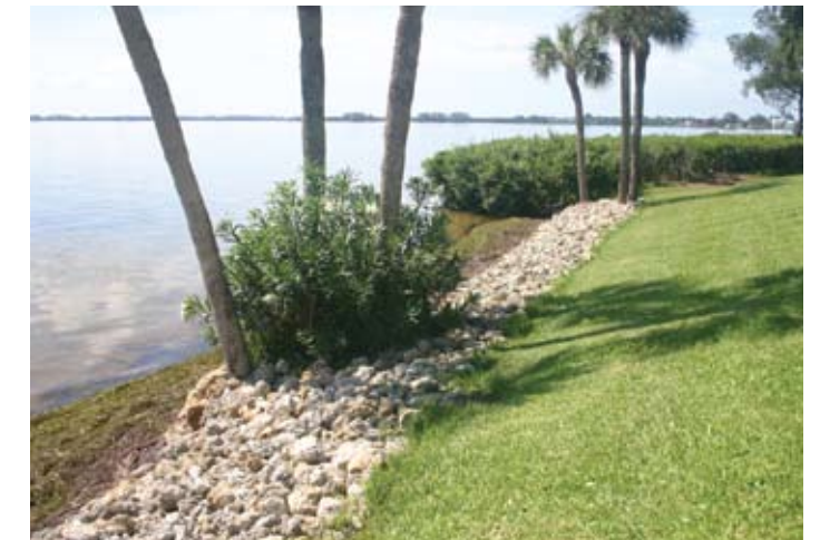
6" – 12" rock installed along graded shoreline
