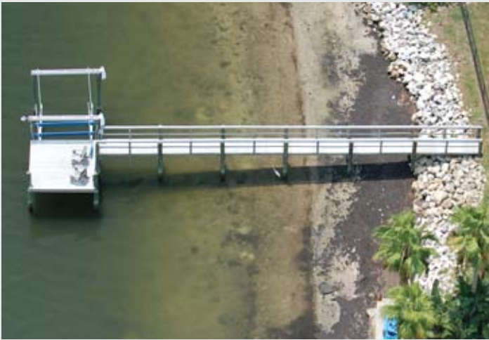
Access and terminal dock with split rail railing, composite decking and 10,000 lb. capacity conventional lift
