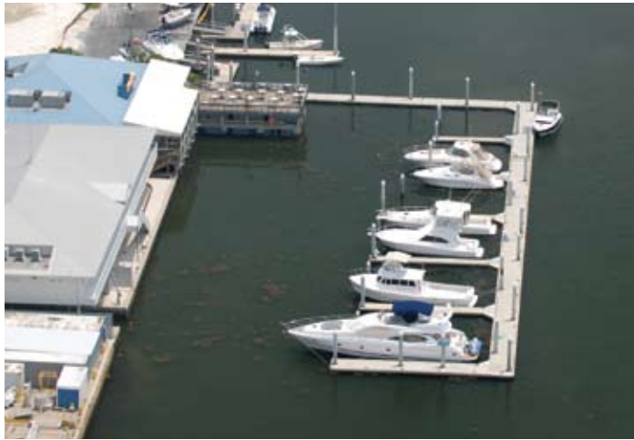
Concrete floating docks installed for Tampa Bayside Marina, Tampa, FL
