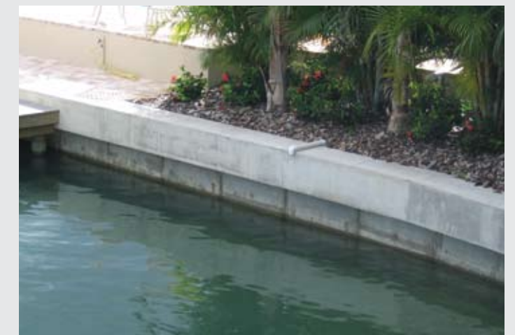
New concrete wall with concrete cap
