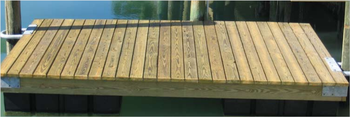
6' x 10' custom-made floating platform
