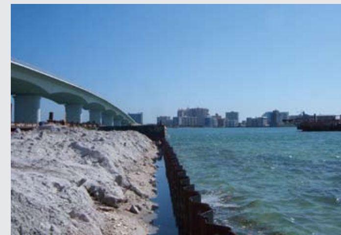
Steel seawall prior to installation of cap at the Ringling Bridge embankment in Sarasota, Florida
