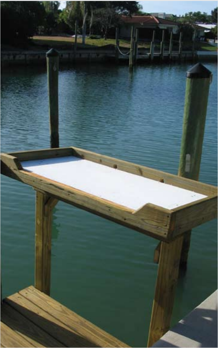
Fish cleaning table trimmed in Pro Deck pressure treated timbers
