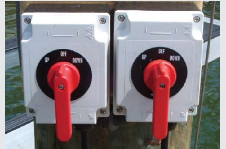
Standard switches for boat lift
