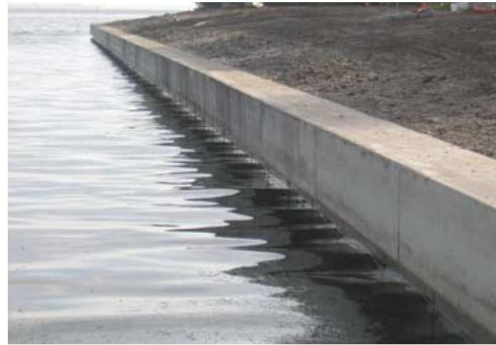
New cap installed on new concrete seawall
