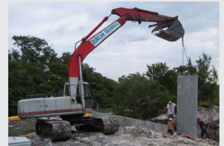
Concrete seawall panel being installed with a land based trackhoe
