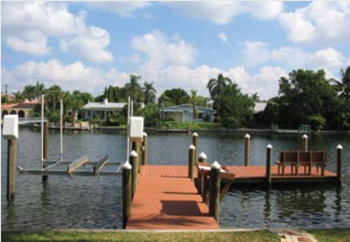
Access and terminal dock with composite decking, 10,000 lb. capacity conventional lift, fish cleaning table, bench and piling caps
